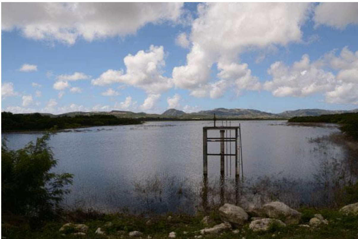
Potworks Dam, check the enlarged steel construction in the species list!
