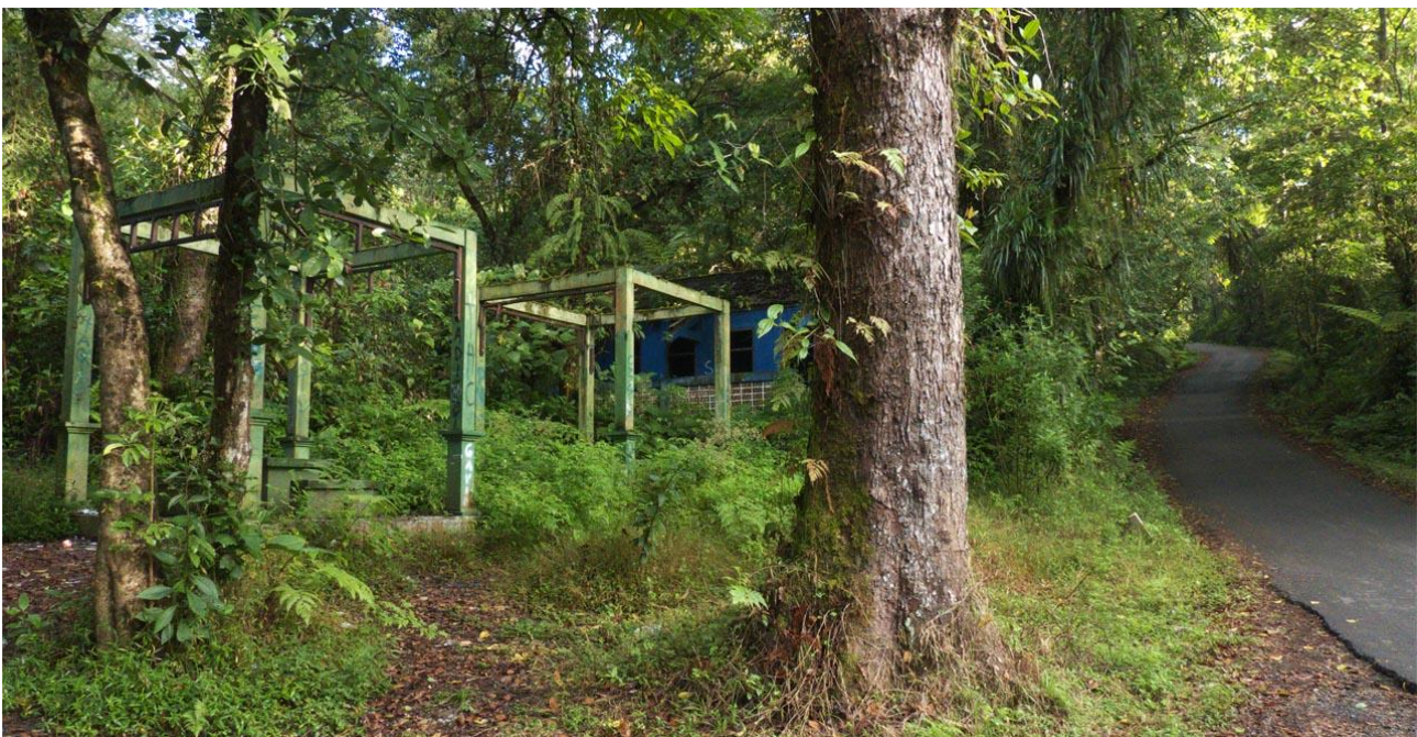
Fig. 11. The derelict Rest Area nr. 2, along the Gunung Ijen access road.
